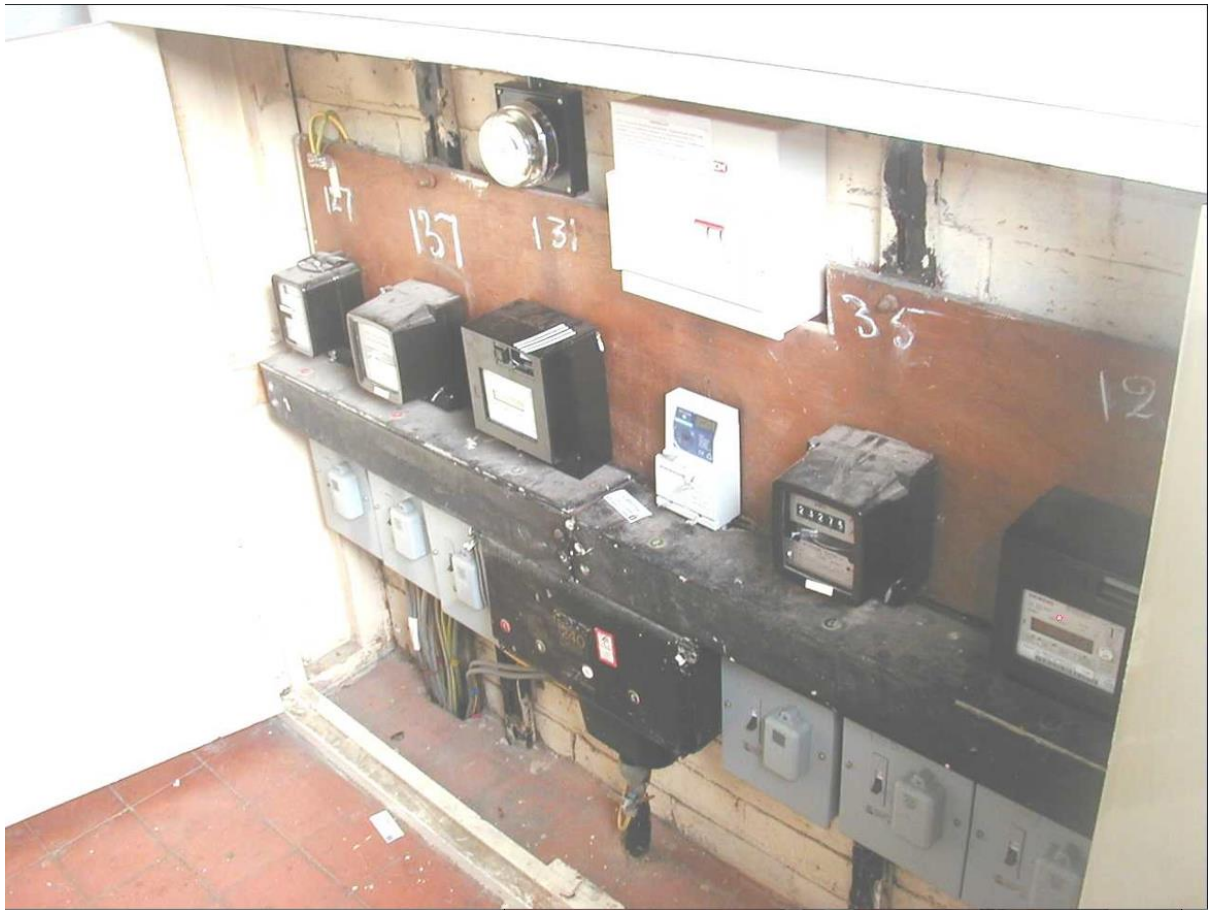
Gas meter sat in asbestos tablet
