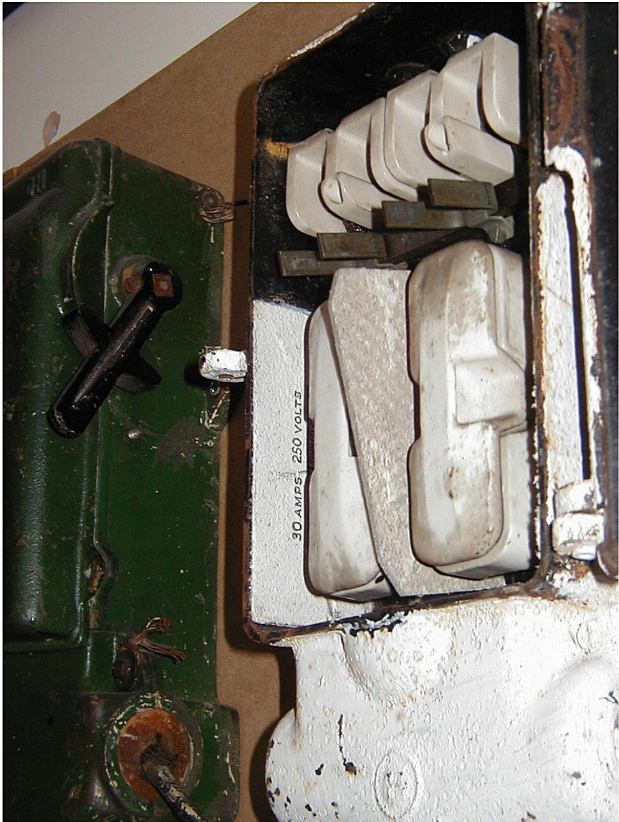
Asbestos divider in cut-out
