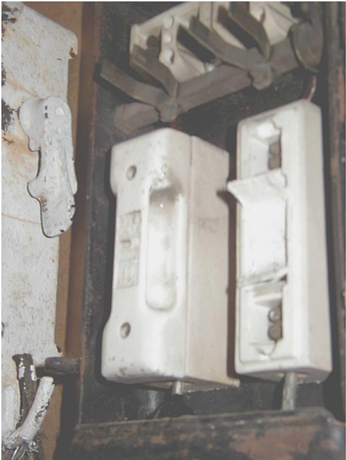
Asbestos Card for fuse suppression
