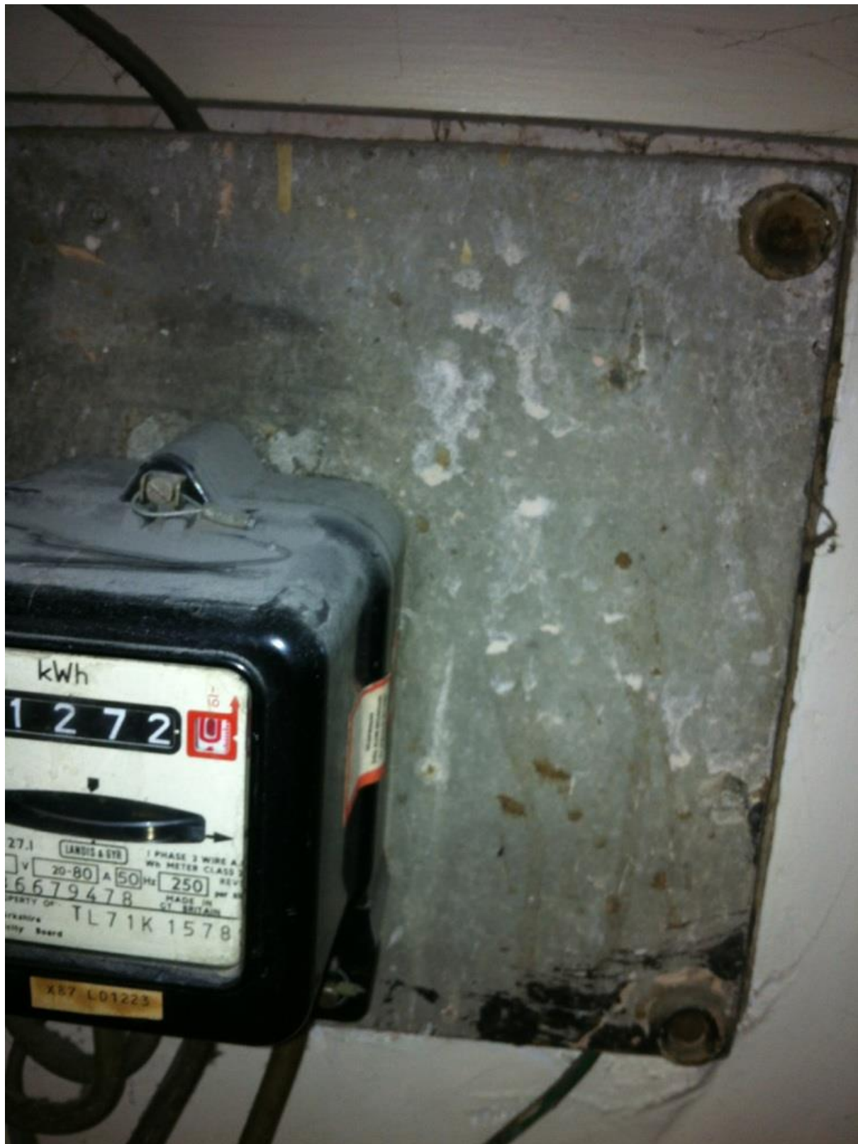
Asbestos Meter Board
